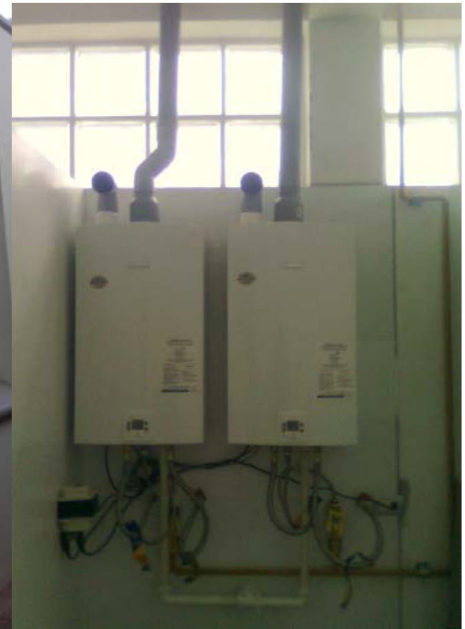
2 x WTD24 in cascading (Indoor installation)
